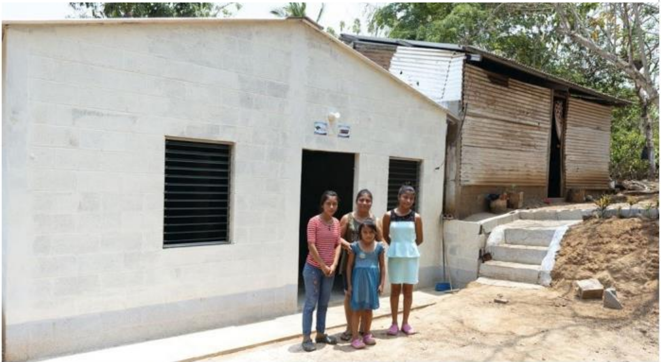
Marleny and her daughters are grateful for their new concrete-block home, built next to their old makeshift home. For the first time, they have windows, a proper door that locks and a cement floor.
