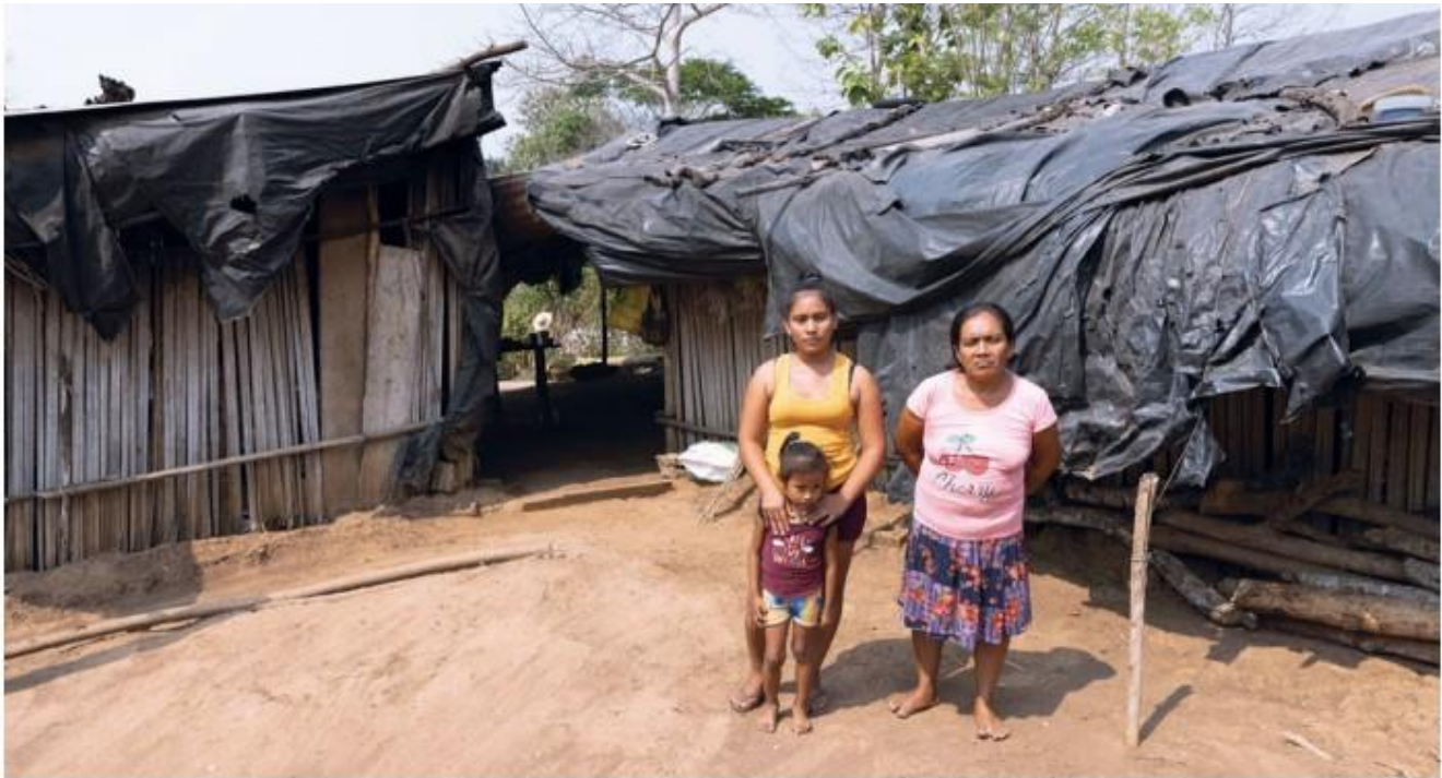
The Morales family places plastic tarps over the thatched roofs of their home and outdoor kitchen to reduce the rainwater that spills inside.
